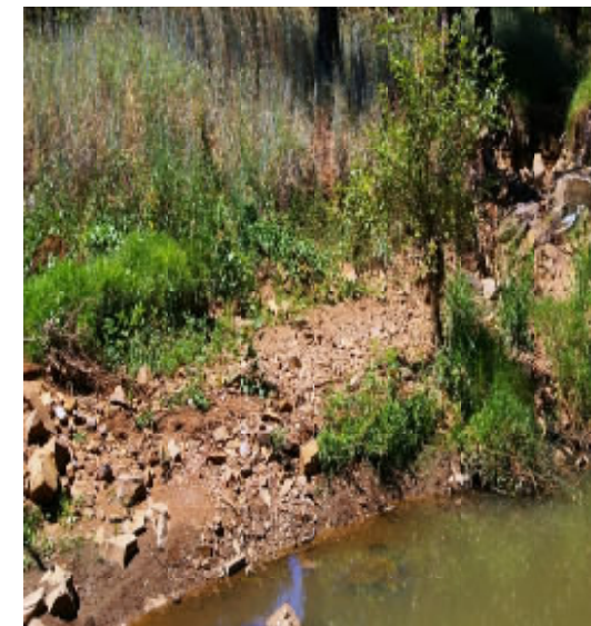
A stretch of riverbank in the Moreleta Reserve showing erosion damage caused by the scouring of the floodwater during the December flood. The loss of vegetation will aggravate the erosion problem during future flooding.
